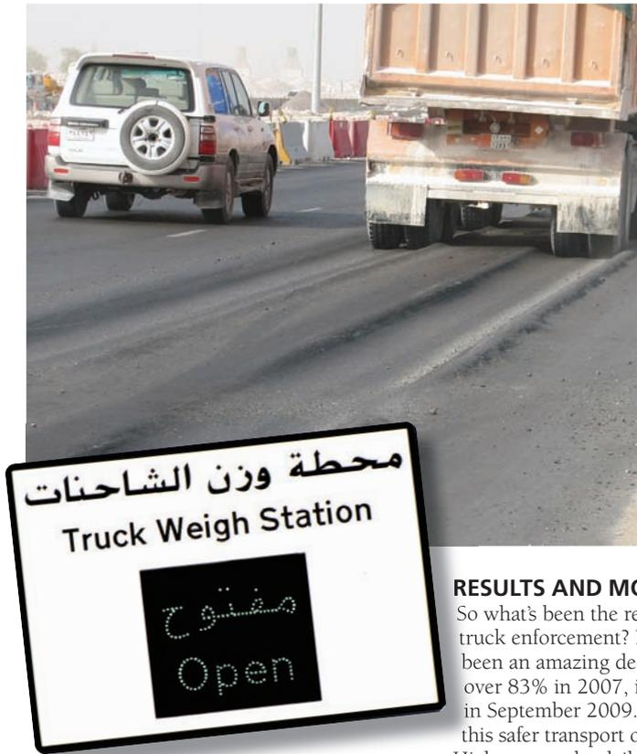
← Showing the damage – severe rutting – that overloaded trucks can cause to roads
