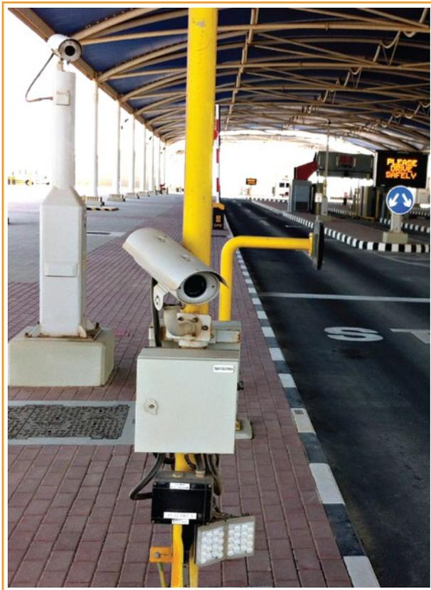
system. The integration was an economical approach as the video feed from the CCTV system is utilized by the ANPR system to capture overview images of each vehicle and saves them as part of the ANPR's transactions. This setup eliminates the need for additional overview cameras for the ANPR.
