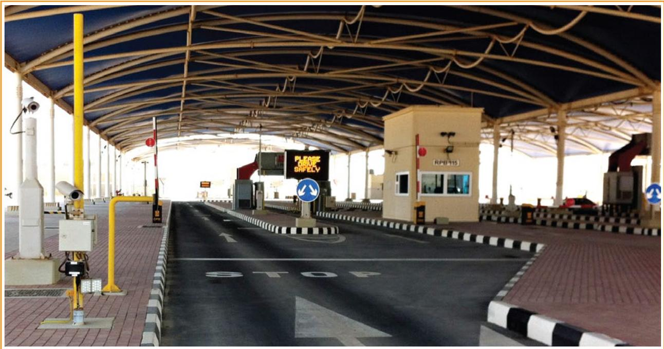
Traffic Tech (Gulf) has completed the installation of 20 lanes of ANPR based Access Control System including Queue-Time Monitoring Module on the two Main Gates of the Ras Laffan Port Expansion Project. The project, commissioned in November 2011, was executed by Traffic Tech through a subcontract agreement with the main contractor, Olive Group FZ LLC.
