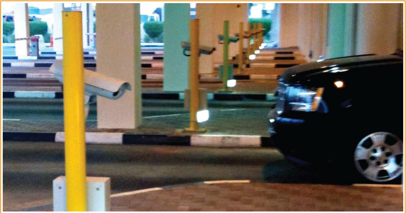
Traffic Tech (Gulf) supplied, installed, and commissioned 18 lanes of ANPR System integrated with iTMS (Intelligent Transport Management System) at Abu Samra, the border that links the State of Qatar and the Kingdom of Saudi Arabia. The system is used by the Borders and Immigration Authority of Qatar to monitor and control all vehicles coming in and out of the country.
